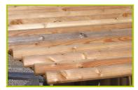
**4- The roofs** are made from larch logs (80 x 40 mm).
