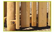
**2- The panels and the climbing wall** are made from larch (plank sizes 140 x 27mm / 45 x 68mm). Larch is naturally resistant and long lasting.
