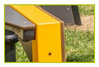
**8- The Central Column seating** is supported by a painted galvanized steel frame structure.
