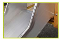
3- The slide is made of stainless steel.
