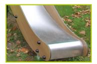
**10-The sliding surface** is made of 2mm thick stainless steel, which is shaped, bent and rolled from one piece.
