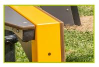
**7- The Central Column seating** is supported by a painted galvanized steel frame structure.
