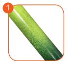
Solid construction made of black steel S235JR ( ø 88,9 - 133 mm), cleaned in the sandblasting process. Protected against corrosion by galvanizing and powder coating with polyester paint QUALICOAT attested.
