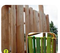
2- The panels, climbing walls, tunnel and beams of the balancing trail items are made from larch (plank sizes  $140 \times 27 \text{ mm} / 45 \times 68 \text{ mm}$ ). Larch is naturally resistant and long lasting.
