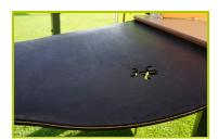
**9- The soft ramp** is made of a woven strip with rubber surface.
