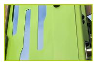
**5- The decorative fence panels** are made of 3mm thick painted aluminium sheets.
