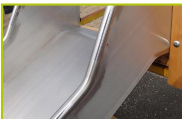
**10-The slide** is made of stainless steel.
